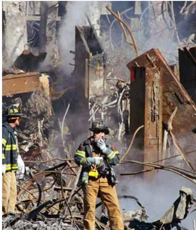
Column showing evidence of a shaped charge having been applied
